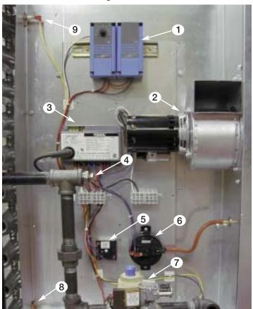
Figure 2: Furnace Control Center
